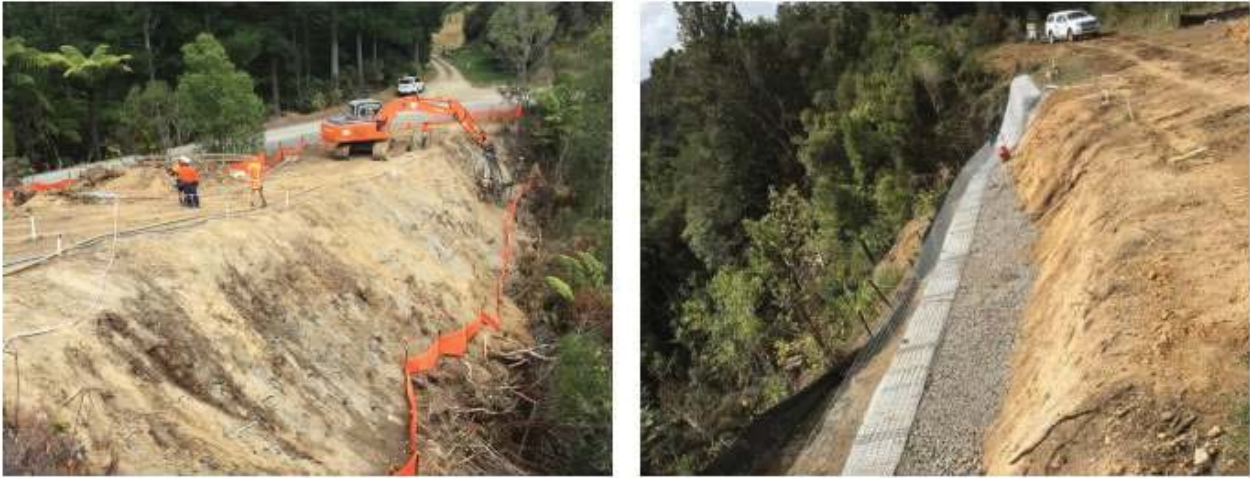
Figure 3: Erosion remediation at Awakau Road
